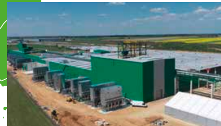
4 Gromadka (PL), Production (under construction)
